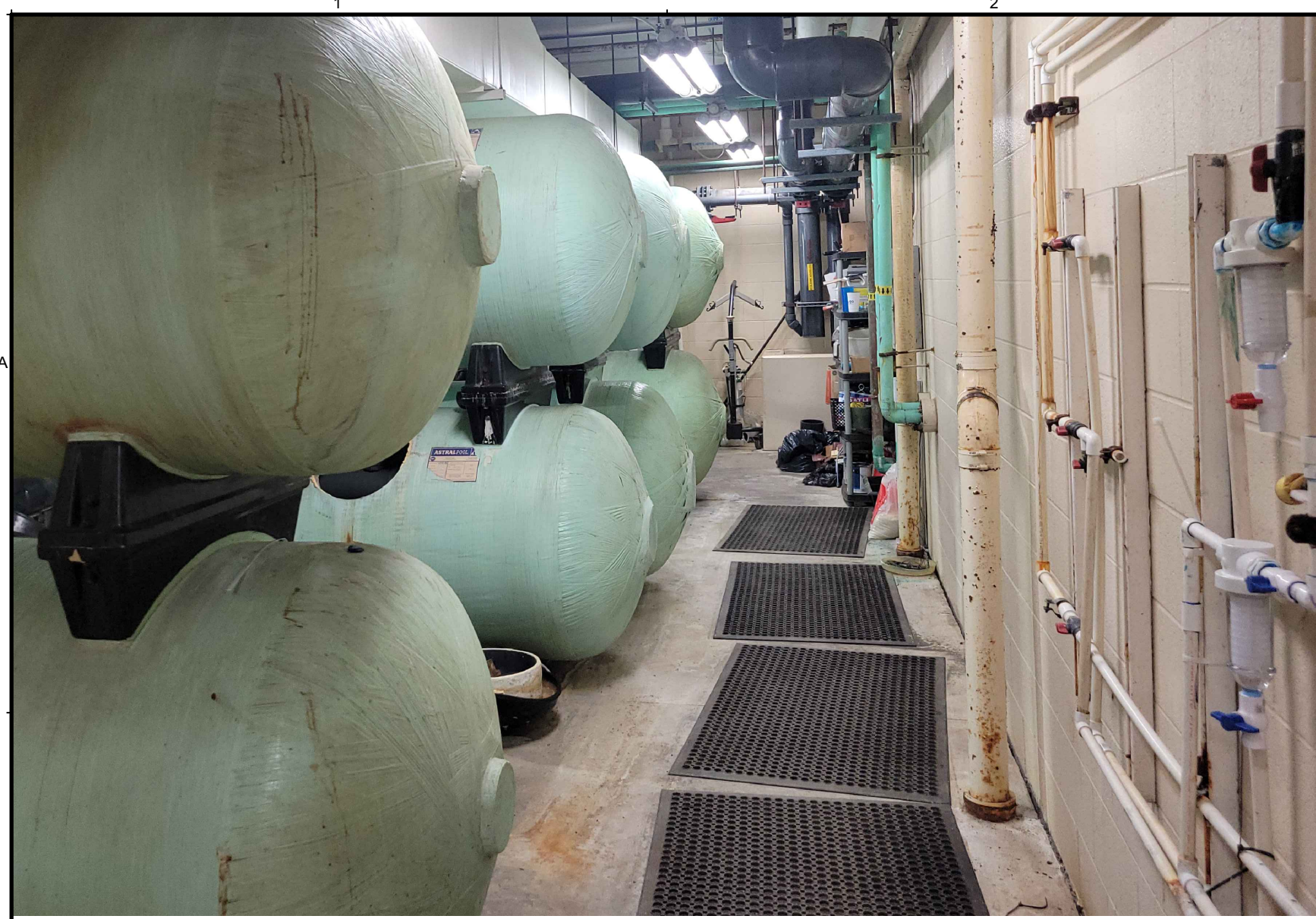
2 EXISTING POOL FILTERS AQ0.02 NTS
