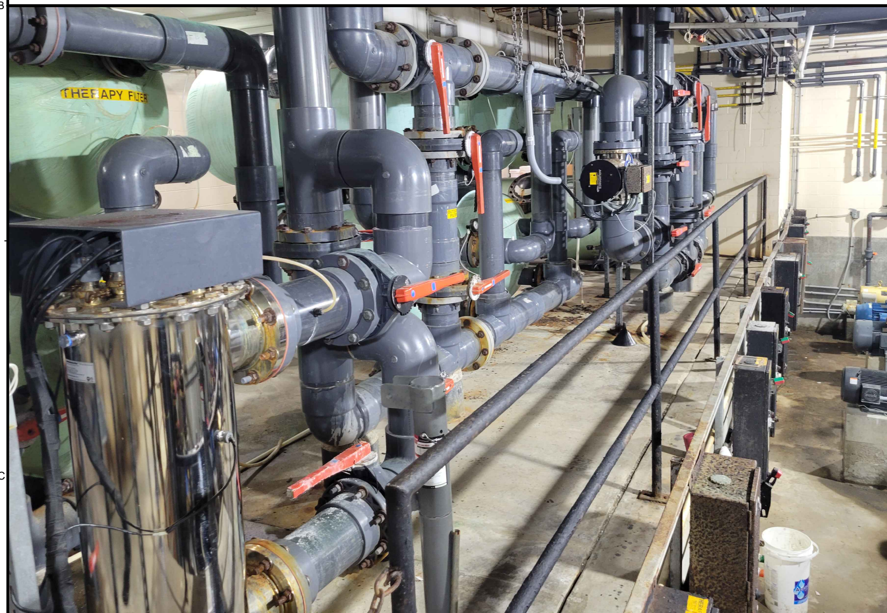
3 EXISTING POOL FILTER FACE PIPING AQ0.02 NTS
